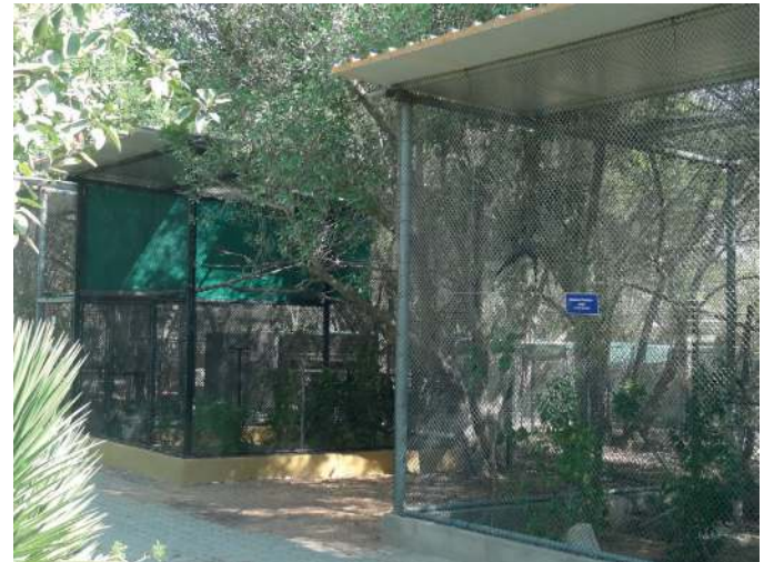
FIGURE 1-4 Painting the cage mesh black creates a “see-through” effect, making the interior of the cage stand out and more visible from a distance compared with an aviary with unpainted mesh. Note the difference between the aviary in the back with its mesh painted black with the one in the front.
