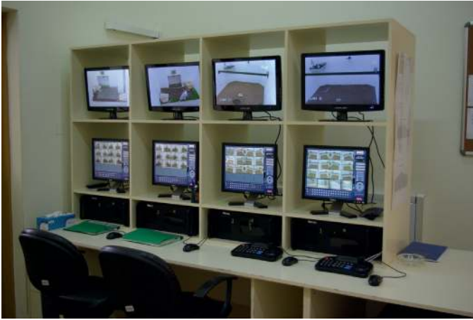
FIGURE 15-5 Video control desk in a modern falcon breeding facility in the Middle East. Two sets of cameras are installed in each breeding chamber. One is focused on the nest; the second, a pan-tilt-zoom camera, allows the operator in the control room to focus and zoom in on different areas of the chamber with the aid of a joystick. Such a system allows video recording, reviewing at different speeds, and retrieving footage of particular interest at any given date for examination. This particular system is also Internet-based, permitting the operator to observe and monitor breeding activity from any locality in the world. (Courtesy Dr. Jaime Samour.)
