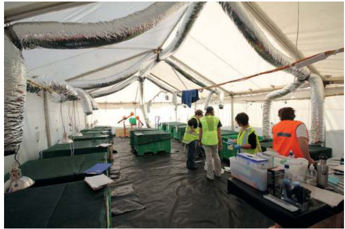
FIGURE 10-43 Thermal support can be provided using a ducted gas system, allowing both heating and ventilation. Heat lamps can provide additional point source heating; however, care must be taken to avoid thermal burns.
