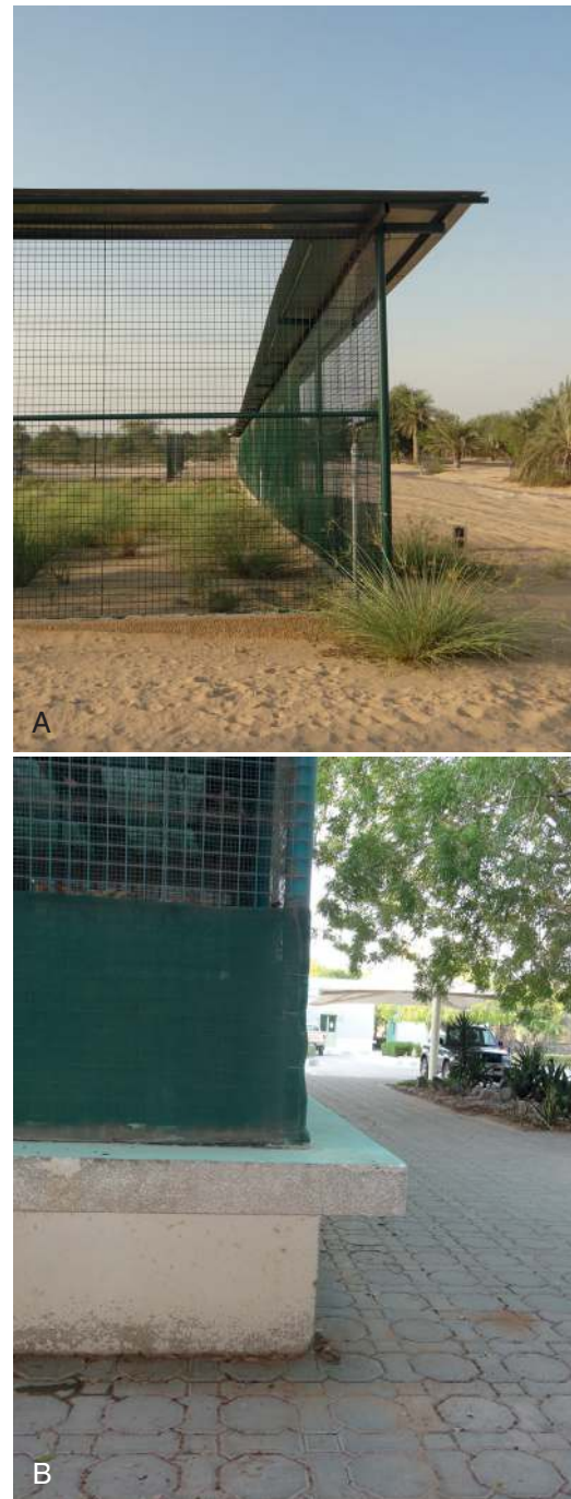
FIGURE 1-9 Aviary designs as practical ways for pest control. (A) , Paddock appropriate for large flightless birds with fox-proofed fencing 3 meters high. (B) , Aviary with rat-proofing 2 feet high at its base.
