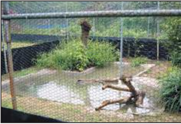
Fig 36.9 | Small concrete pools are easy to clean and maintain.
