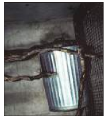
Fig 1.11e | Rodents leave a black streak from body oil on the wall over this perch in the cockatoo facility of a prominent US zoo. The heavy stain indicated a lack of effective pest control measures.
