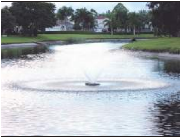
Fig 36.11 | Water aerator for a large pond.
