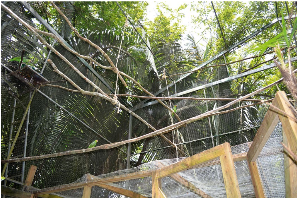
Figure 39.8 Box steel 2×4 primary supports in a very large aviary, with a variety of ropes and perches.
