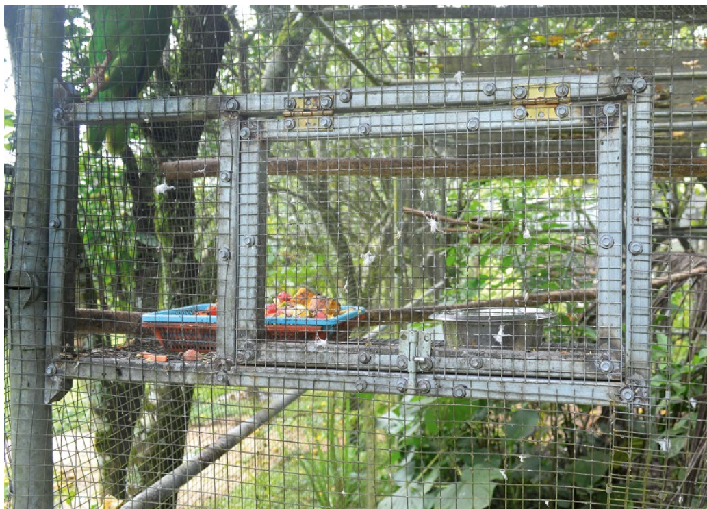
Figure 39.4 Double plate system for food trays and a stout water bowl, with a wall hatch that allows food delivery without direct interaction with the birds.
