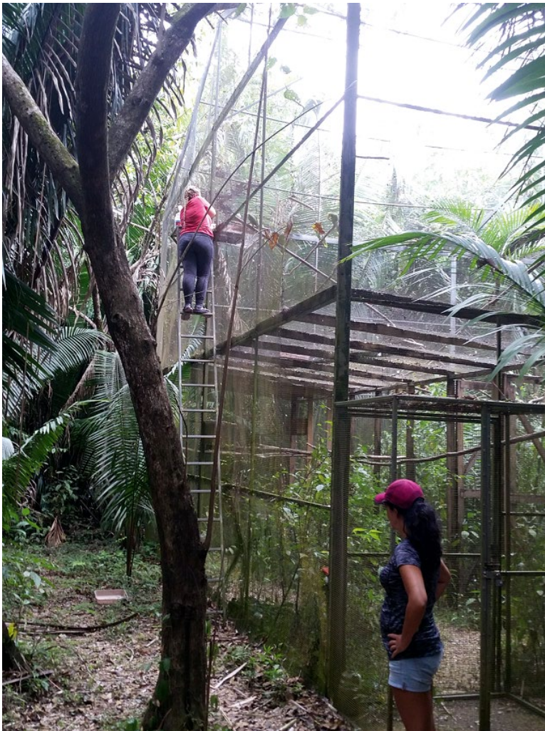
Figure 39.6 A large footprint, tall aviary is needed for pre-release activity and social interaction. Note the hatch that allows feeding at elevation.
