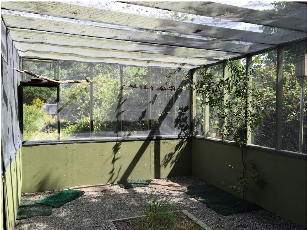
Figure 44.7 Swallow aviary: large open space in the middle to support unobstructed flight path and room to maneuver, perching options at the end include rope and natural branches, elevated shelf to hold water and food dishes, AstroTurf mats are placed directly under perching areas to facilitate easy clean-up of feces.
