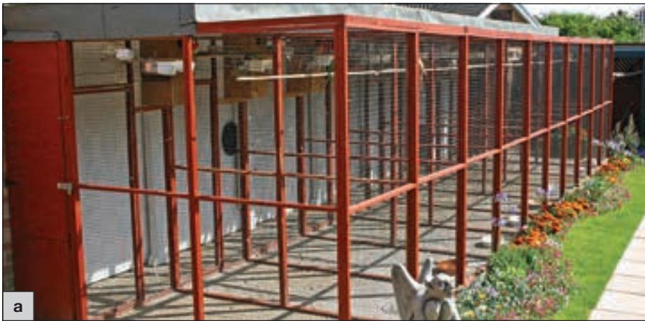
3.3 The three-thirds aviary setup. (a) A wooden-framed garden aviary for small parakeets, showing a door to a rear service corridor; a row of flights, each with a nest box and feeding dishes under the felt roof; an open section of flight with a perch to allow the birds access to sun and rain; a sloping floor of paving slabs for ease of cleaning and large shallow water dishes for bathing. The whole unit is incorporated into the garden as an attractive feature. Note that this aviary is not double-wired, thus leaving the birds vulnerable to predator attack.
